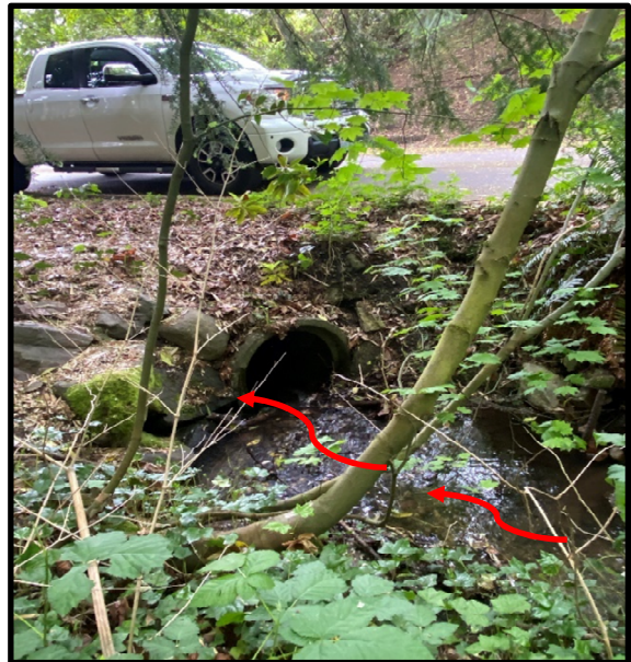
Point – 14 , Surface flows enter an existing 24" concrete culvert.
