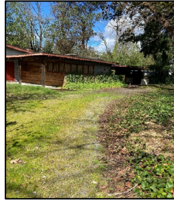
Pic-4 , looking NW at existing house
