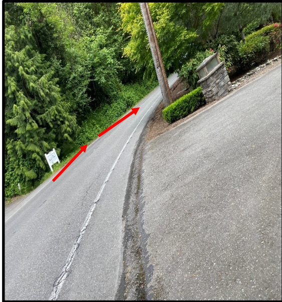
Point – 11 , Surface flows continue in natural drainage channel.
