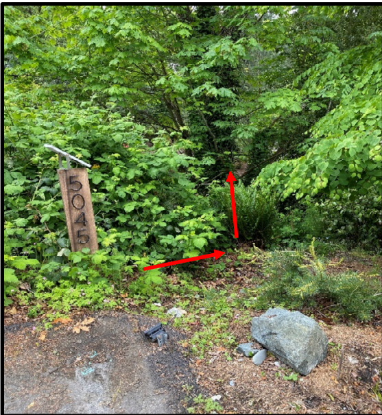
Point – 9 , Surface flows discharge in existing natural drainage channel.
