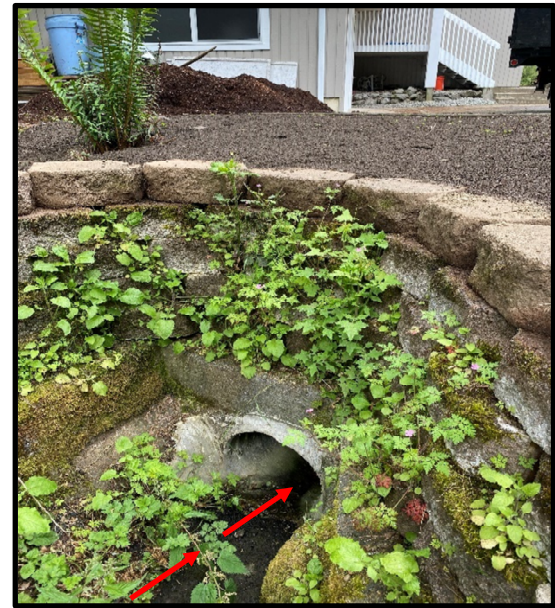
Point – 6 , Surface flows enter Ex. 18" Culvert
