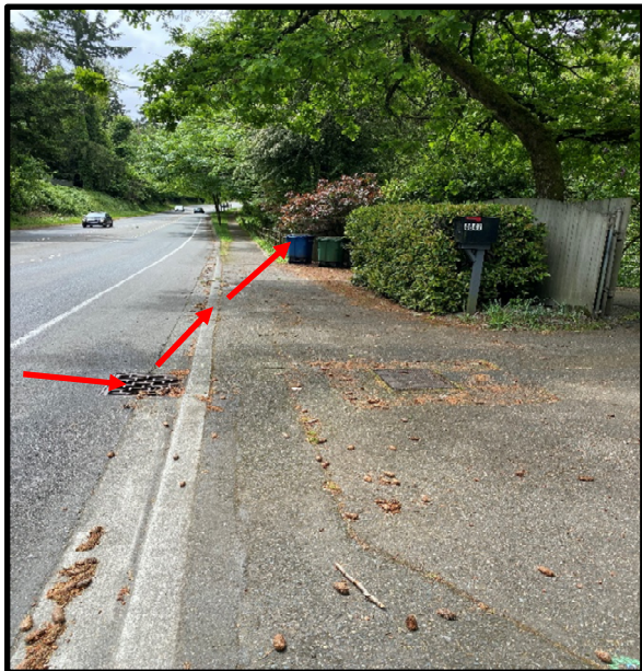
Point – 3 , Surface flows enter existing CB on west side
