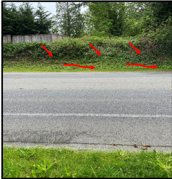
Point – 1A, Surface flows leaves the site in sheet flow Island Format.
